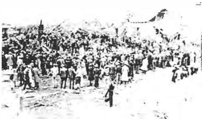
Many people were injured or killed when the tornado hit. Many were lost to their families and had to be searched out from the rubble.
